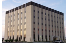
UEI Headquarters Houston, TX
