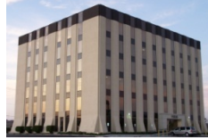
UEI Headquarters Houston, TX
