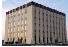
UEI Headquarters Houston, TX
