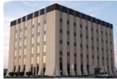
UEI Headquarters Houston, TX
