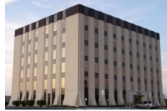
UEI Headquarters Houston, TX
